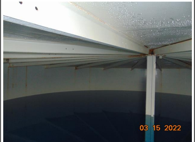
17) Rafters and center column
