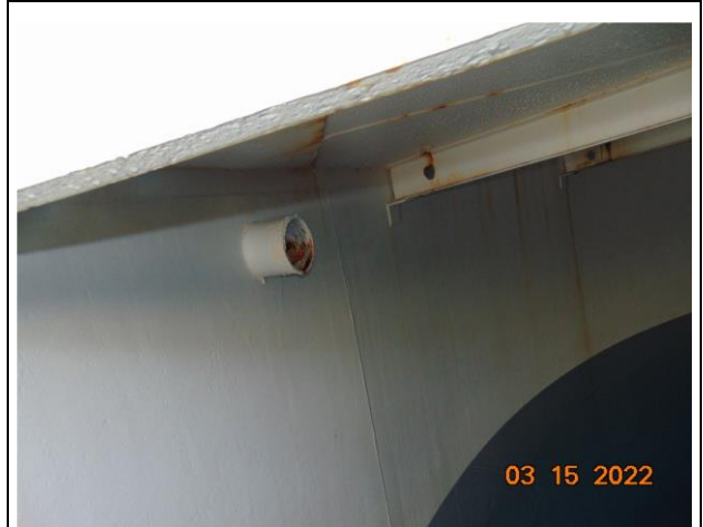
16) Overflow pipe and shell
