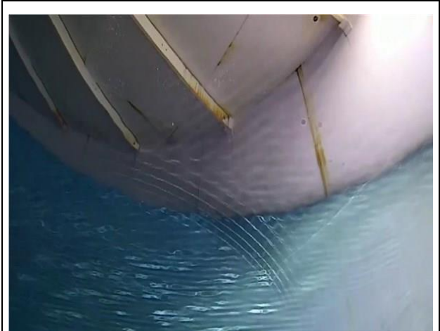
22) 00:37 Roof to shell seam
