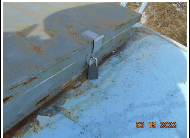
18) Locked roof hatch
