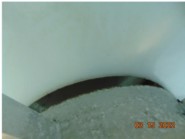
14) Vent vacuum plate warped
