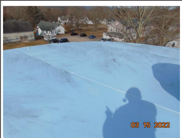
10) Typical condition of roof plates
