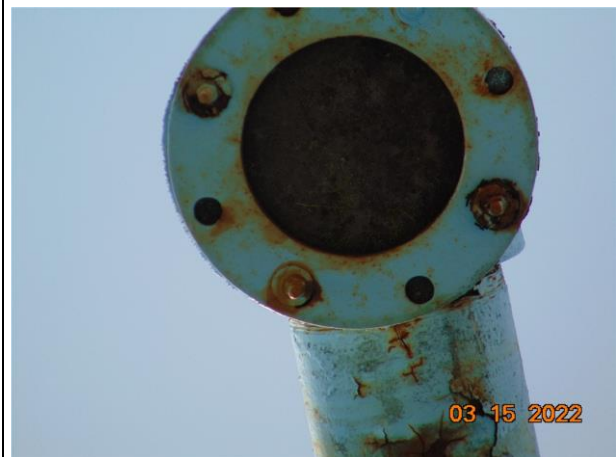
20) Intact overflow screen
