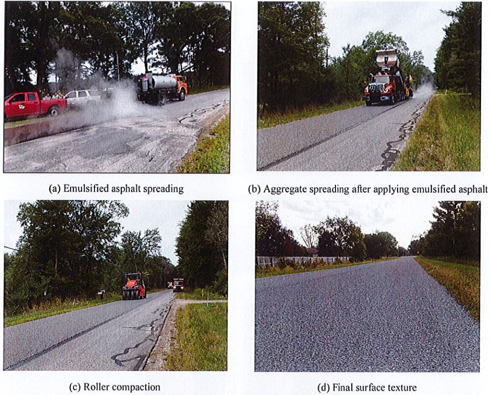
Fig. 12. Asphalt emulsion chip seal construction process.
