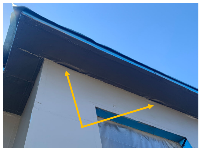
Examples of air bubbles or voids below the fluid applied membrane.
