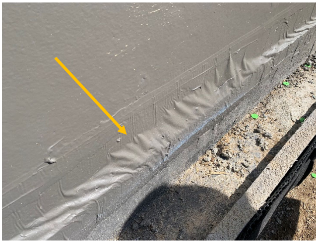
Examples of air bubbles or voids below the fluid applied membrane.
