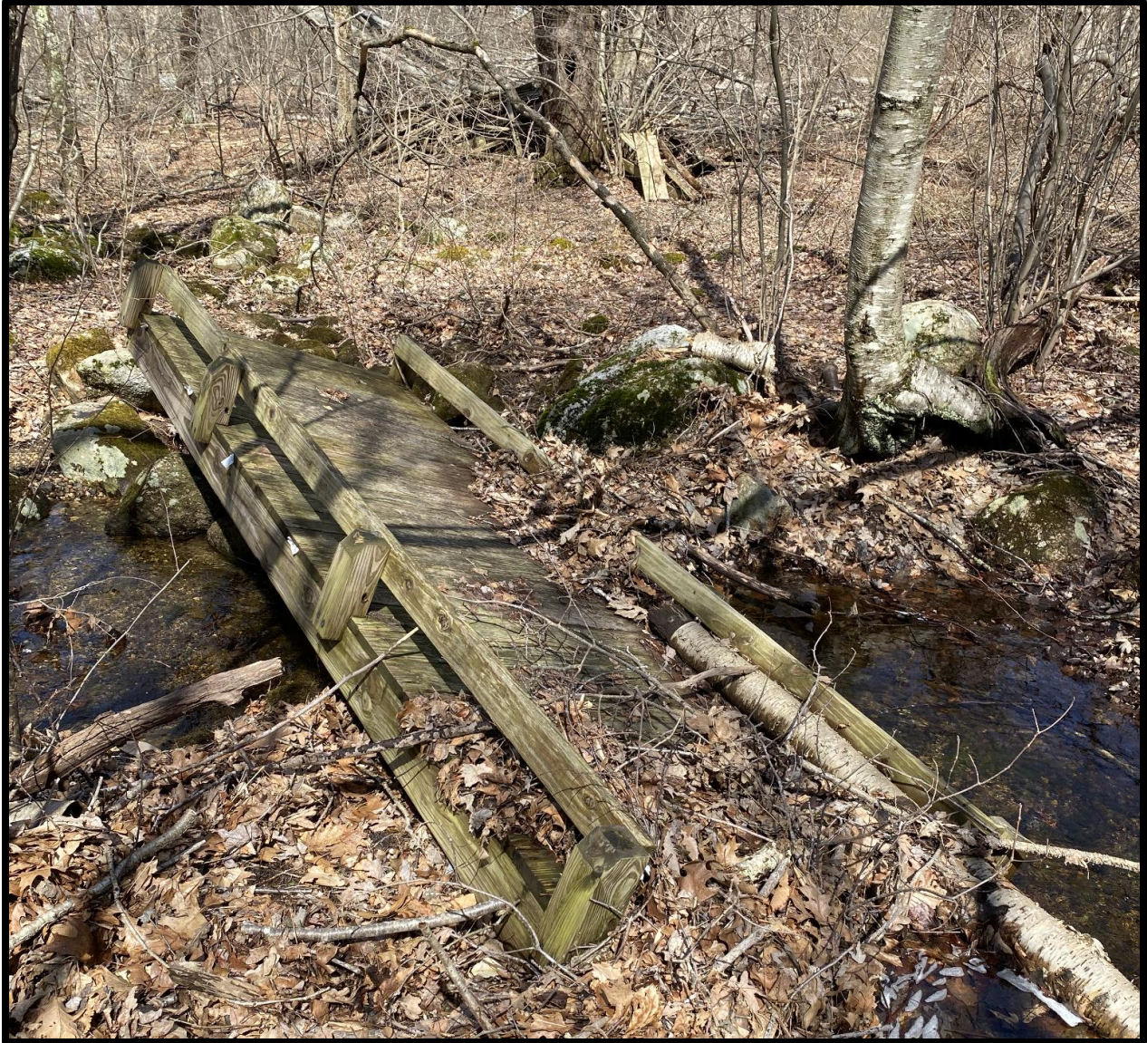
Figure 25. Image of washed out footbridge on southern end of the red trail - an example of the damage and debris making some of the trails difficult to use at Ruby Cohen. (Source: Jamie Kurowski)
